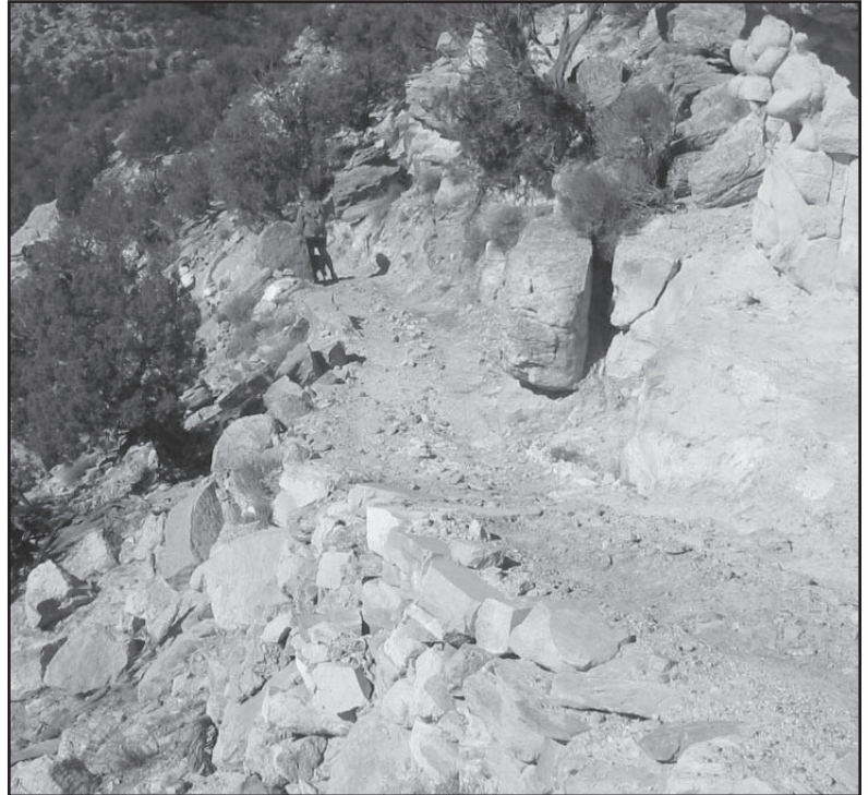
Cribbing/fill constructed along the cliff face of the Recapture Wash route allows new ATV access where it was previously impassable.
