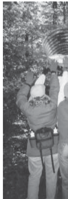
Now, it's up, up, and a... culvert. Photo by Ann
