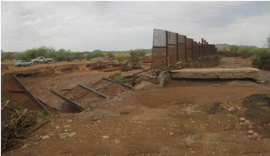
Border in Organ Pipe Cactus National Monument washed away in 2011. National Park Service photo.
