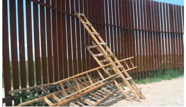
LADDERS ACCUMULATE ALONG A BOLLARD BORDER WALL IN TEXAS. PHOTO: SCOTT NICOL
