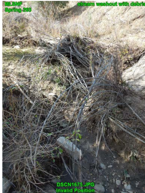
Fig. 3: Debris in the streambed
