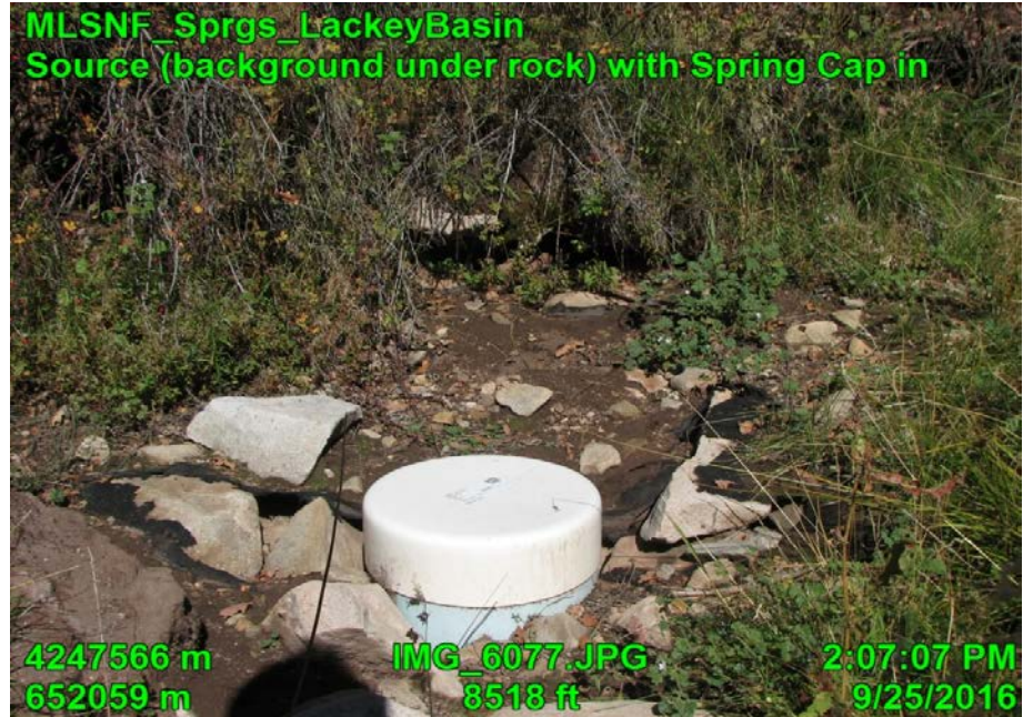
Fig. 1: Source beneath rock (top center), w/ capped spring containment in foreground
