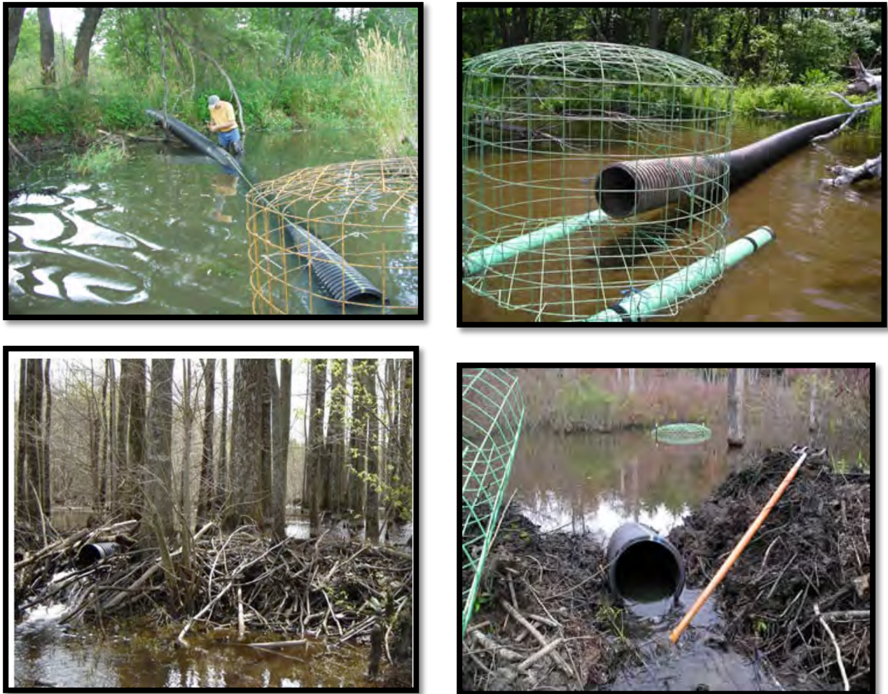
Figure 40: Flexible pond levelers with cylindrical wire cages on the upstream pipe end. Clockwise from upper left (a) and (b) are examples during the construction phase, while (c) is an example just after completion but before dam repair. (d) is a downstream view of a pond leveler after beaver have repaired the dam. Photographs from Boyle (2006).
